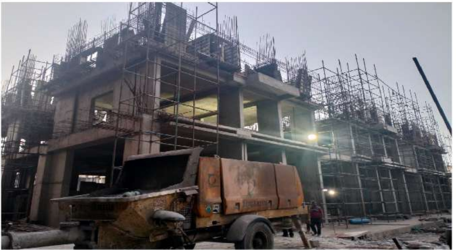
TOWER 1 :: SLAB AT 3 rd FLOOR LEVEL IN PROGRESS
